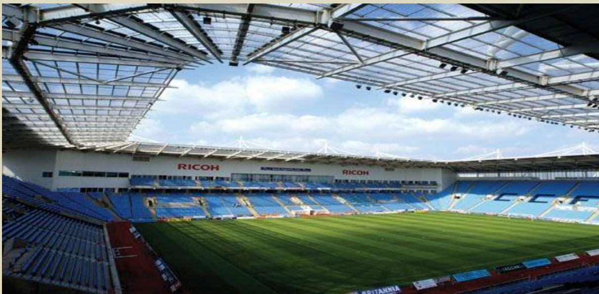
South, West and North Stands
